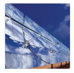
The use of solar energy to generate heat requires a suitable transfer medium to transport the heat generated. Various media, which are primarily based on water and oil, are used for this purpose. Maximum heat transfer leads to high system temperatures and therefore makes extremely high demands on the sealing materials used in the connecting elements of the transfer system.
