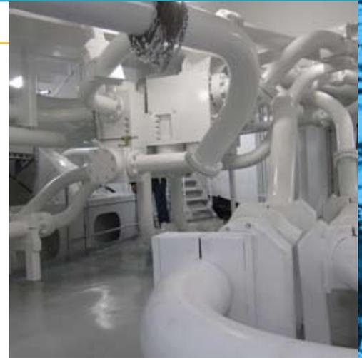
Parker recently worked with one of its customers on one of the most advanced diving support vessels in the world. Parker's non-welded solution for the vessel included 190 x 20 mm (7.5" x .8") pipe spools, which reduced flushing time by 50 percent, provided system pressure of 350 bar (5,076 psi), and produced zero leakage at start-up.
